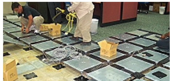
Camass installed on top of old embed floor trunkings renovation proceeding, and office in normal operation
