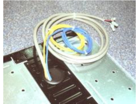
Cables extending from cable trenches to workstations or partitions
